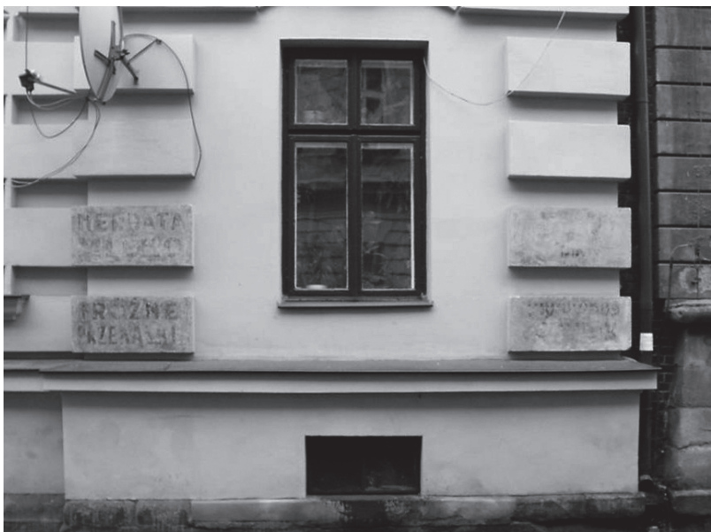
Photo 2 Second Facade of the building at ul. Goldhammer (2000)
